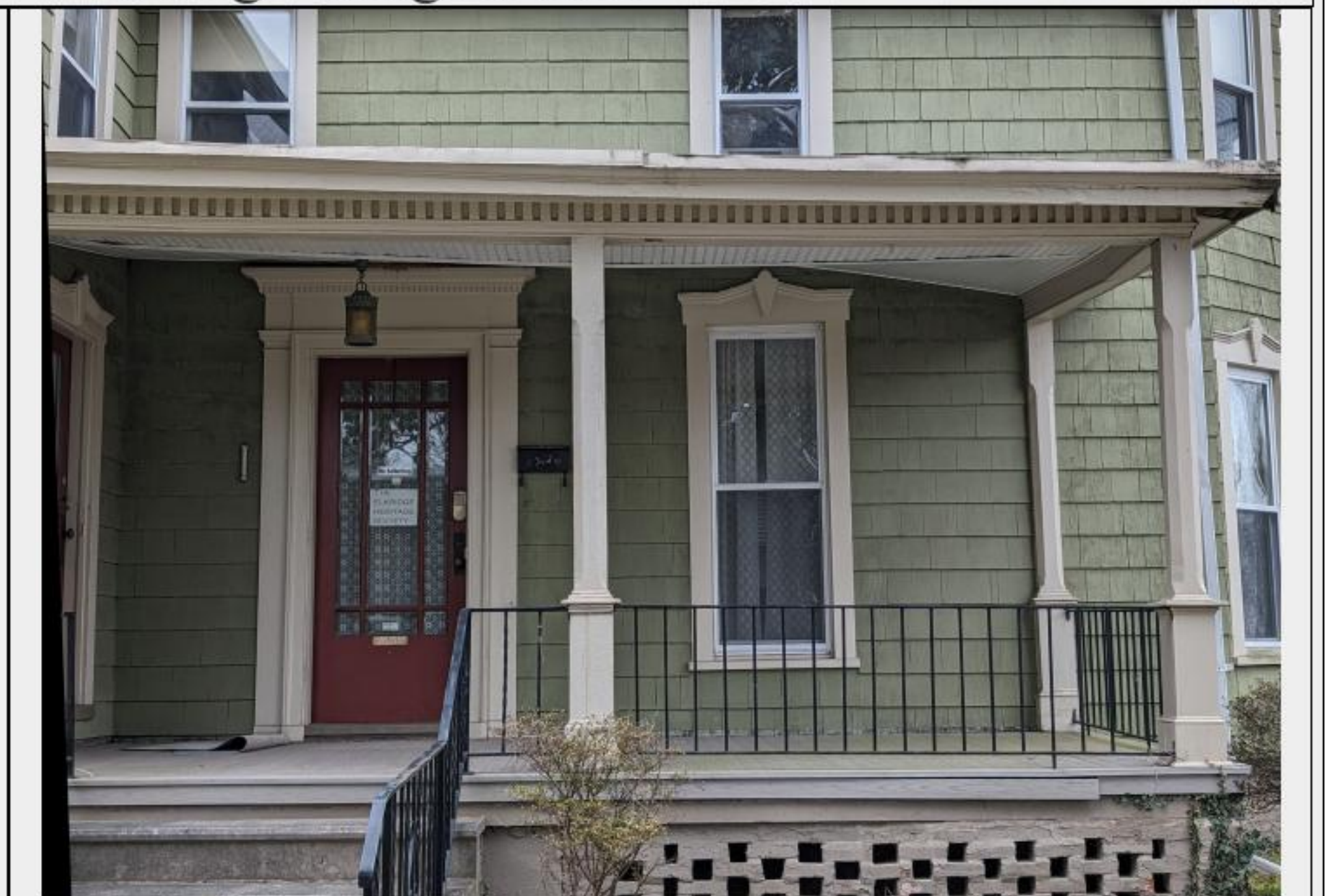
Porch was renovated in 2019, except roof
