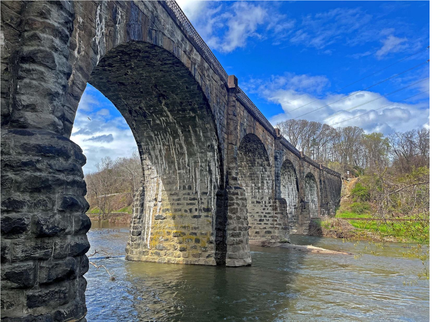
East Side looking North, April 2024
