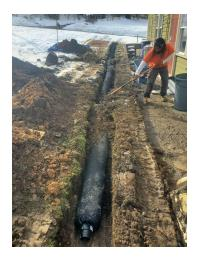
Meanwhile, we contacted a company to assess the water problem in the basement. We had to get some brush cleared and have a French Drain installed due to the way the lawn slopes into the back of the house. (See the photo, left.)
